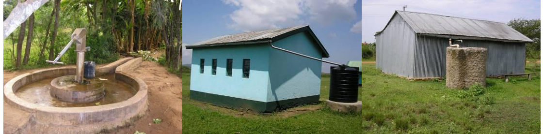
Pic. 3, a shallow water well. Pic.4 water harvesting in an administration block of a local primary school Pic. 5 water harvesting in a local rice milling structure
